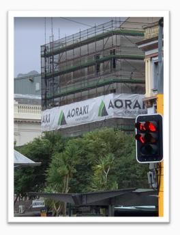
Work includes re-strengthening the existing structure via new foundations and concrete shear walls. Existing windows will be replaced, and the interior apartments will "make great use of the building's 1934 deco-era charm!". More info/pix here
