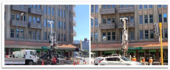
There was a drilling machine working on the corner of Taranaki Street and Wakefield Street. When asked, the man in the hard hat with the clipboard seemed to indicate they were drilling to check on the nature of the ground in that spot.
